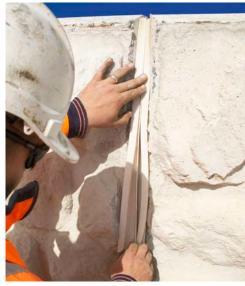
The ELASTOSIL R® silicone rubber used in the Boss SpineSeal on the EastLink freeway sound barriers is UV, heat, ozone and weathering resistant. Proven in tests, including climate DIN50018-SW2.0S and ozone DIN53509-1, it is designed to deliver life of 30-plus years
