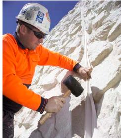
Boss SpineSeal – installed in sound barriers on the EastLink freeway – is an extruded rubber fin shaped seal, which is folded over a rigid backbone, and then driven into the gap using simple hand tools.
