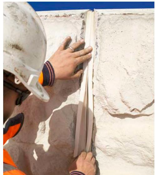
The ELASTOSIL R® silicone rubber used in the Boss SpineSeal on the EastLink freeway sound barriers is UV, heat, ozone and weathering resistant. Proven in tests, including climate DIN50018-SW2.0S and ozone DIN53509-1, it is designed to deliver life of 30-plus years.
