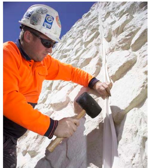
Boss SpineSeal – installed in sound barriers on the EastLink freeway – is an extruded rubber fin shaped seal, which is folded over a rigid backbone, and then driven into the gap using simple hand tools.
